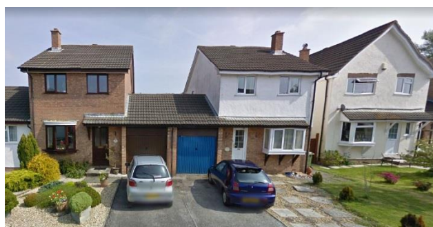
Photo 11: Example of properties on Dornafield Drive East
