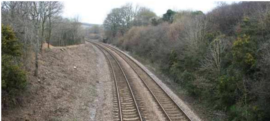
Part of the mainline railway
